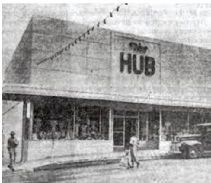
The Hub while in Operation
