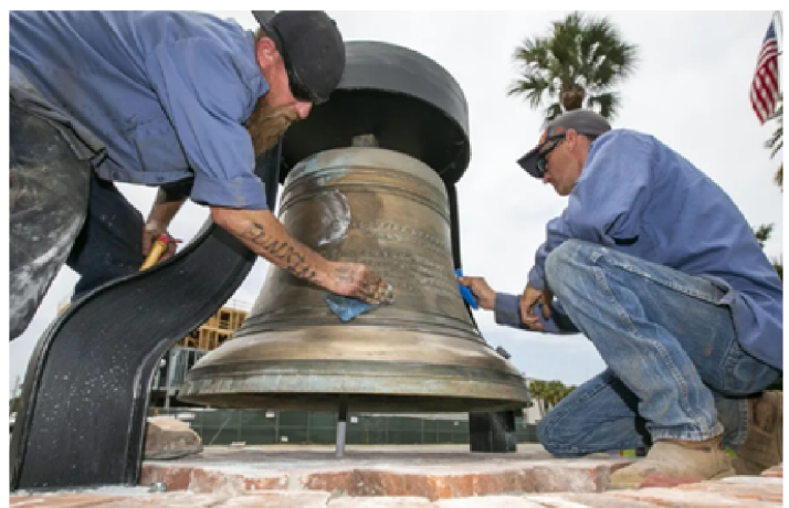
Bell Being Re-Installed Downtown
