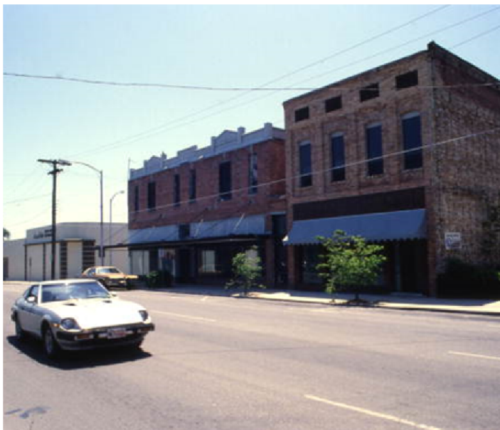
Hood Block (right brick building) c.1970
