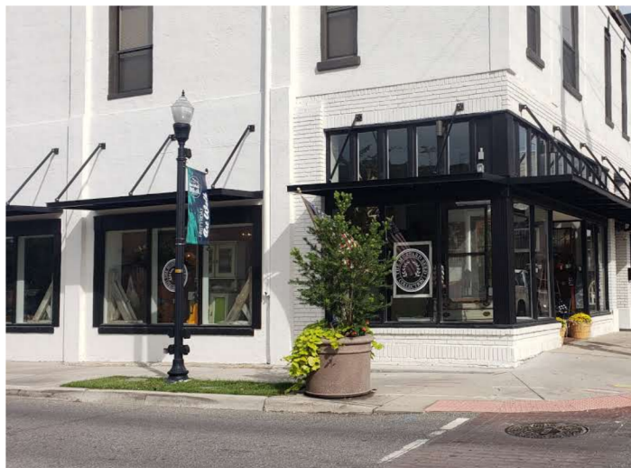
Banner Block renovated, 2022
